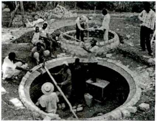
Fig. 1b: Fixed-half-dome digester design
