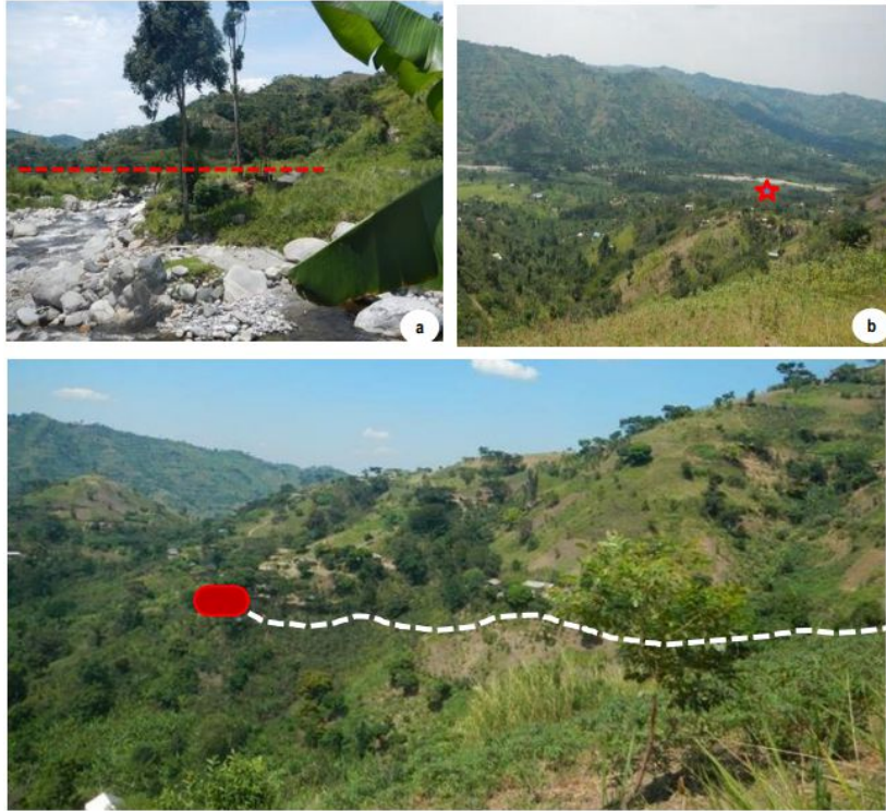
Plate 1. (a) Location of Nyamughasana-2 HPP intake weir (red line in middle ground was constructed). (b) Location where construction was done for the power house area (red star), seen from fore bay on right side of Nyamughasana River in a relatively flat area. (c) Proposed location of fore bay (red box) and approximate proposed location of canal (dotted line).
